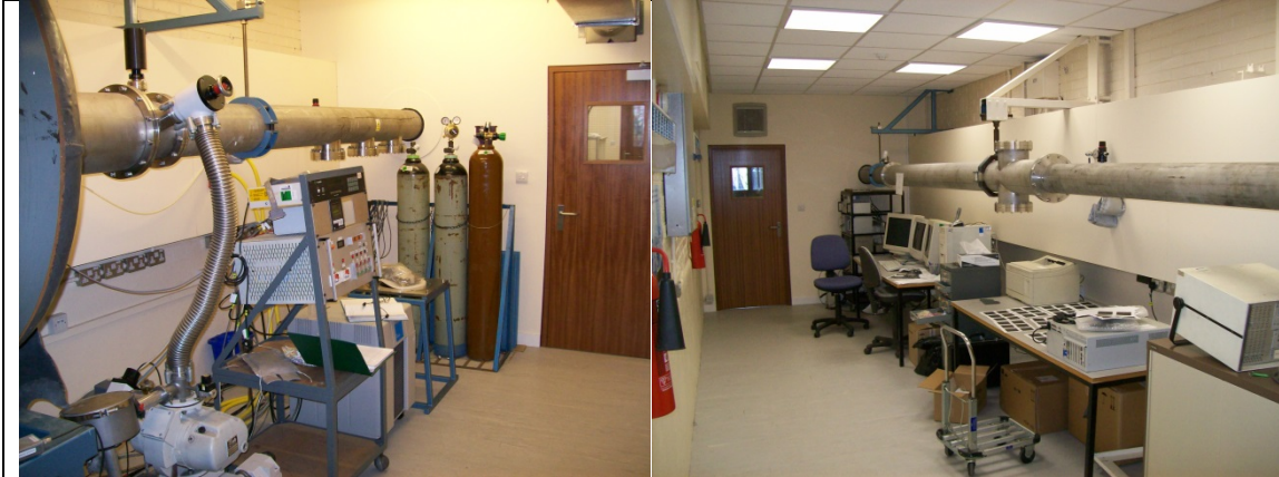
Figure 4: Vacuum area showing 3 beamline access points
